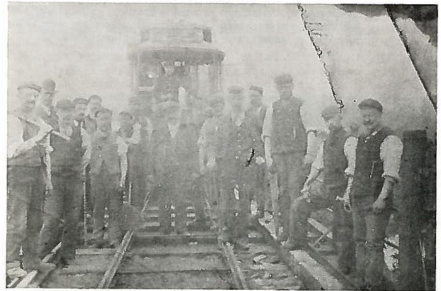
Top: Permanent way gang at work on changing the bull head rails for the grooved girder tramway rails.
